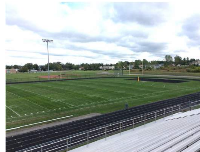
EAST SENIOR HIGH SCHOOL Construction 2020
